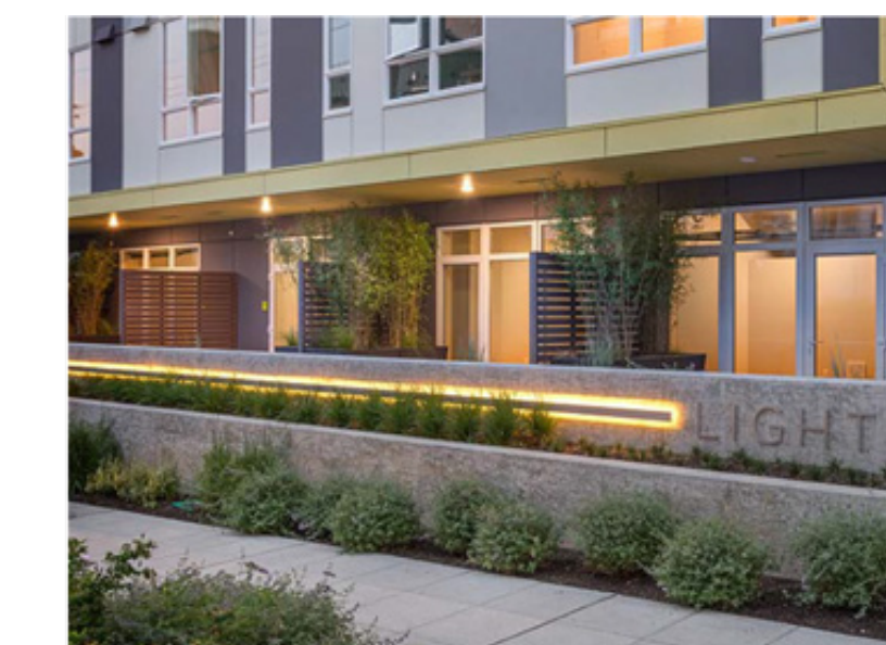
Raised terraces provide some privacy and while engaging the street.
